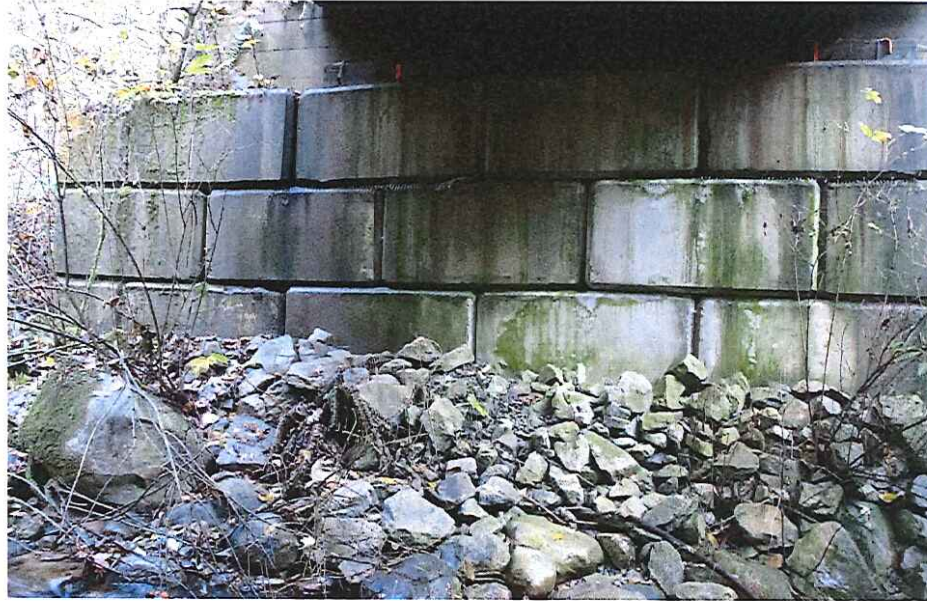
CK2012 Left Abutment
