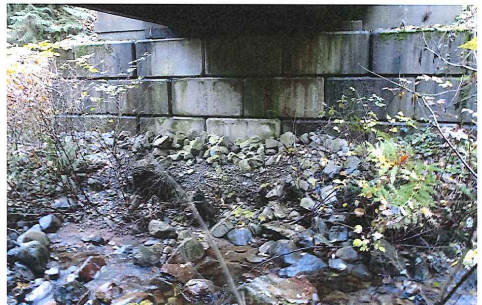
CK2012 Right Abutment
