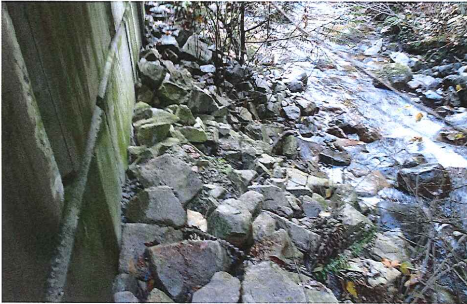
CK2012 Left Abutment rip rap
